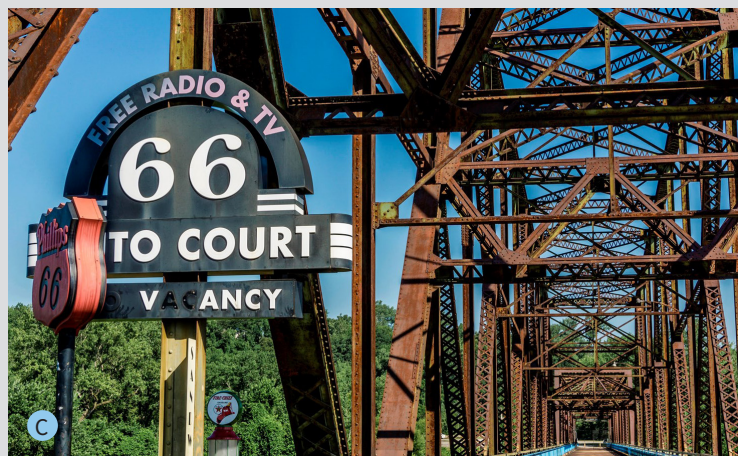
Chain of Rocks Bridge from Madison, Illinois, to St. Louis, Missouri
